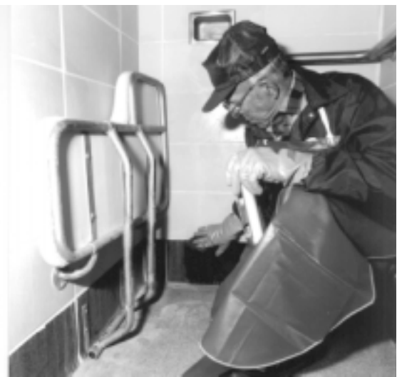
Mineral deposits and soap scum can be removed with a scale remover. (NOTE: In some locations, treating the water by installing a water softener system can greatly reduce the mineral deposit)
